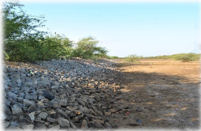
A poorly constructed seawall in Ngomeni, Malindi
